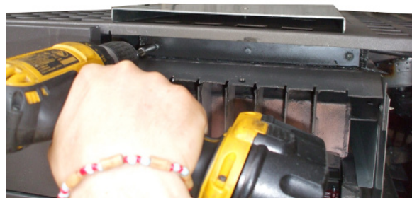
Fig. 54 - Remove top cover
