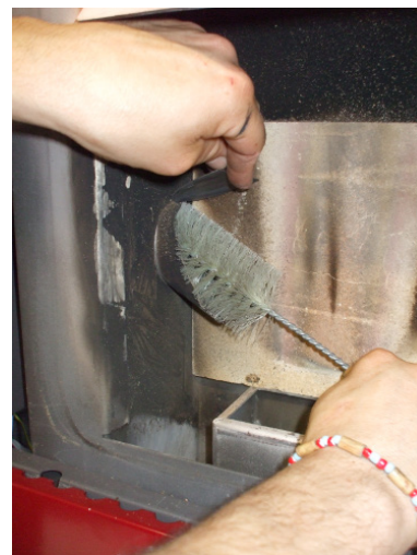
Fig. 44 - Cleaning with a brush
