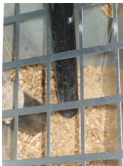
Fig. 45 - Hopper and auger cleaning
